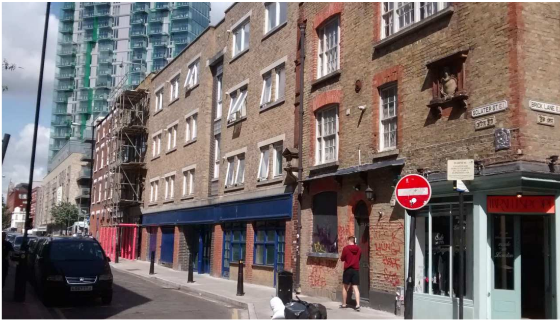
4.5 Site (behind scaffold) and terrace of properties along Sclater Street.
